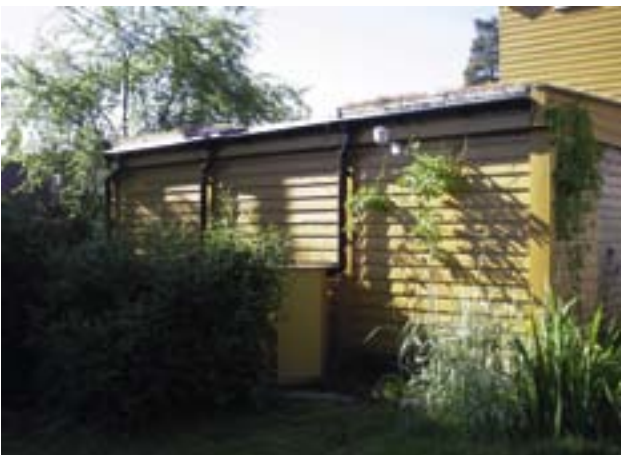
Green vegetative roofs
