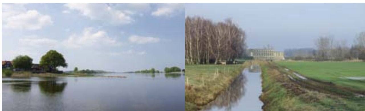
Left: River Elbe Right: Pumpig Station
